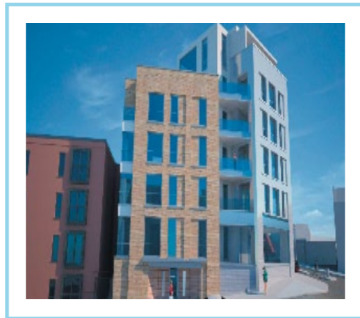
355 Ladbrooke Grove, W10. 9 Apartments under construction
