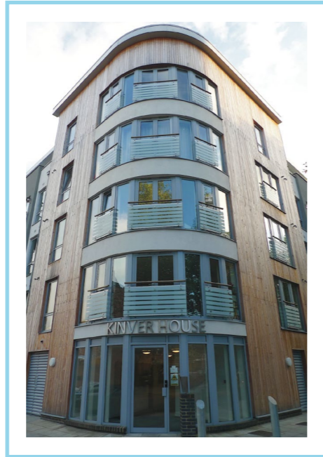
Kinver House, Archway, N19. 85 Apartments
